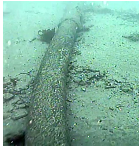
Figure: Submerged pipeline laid on seafloor
